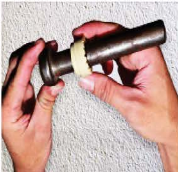
INSERTING OF CERAMIC INTO STUDS
