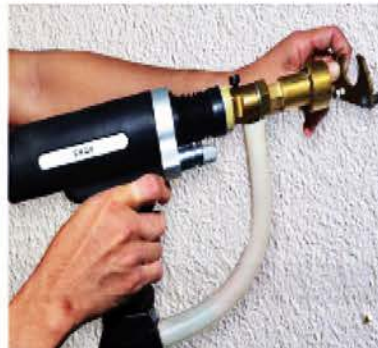
ALIGNING THE STUD PROPERLY ON THE METAL SURFACE
