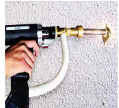
SPLIT-SECOND STUD WELDING INSTALLATION
