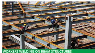
WORKERS WELDING ON BEAM STRUCTURES
