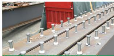
STUDS INSTALLED ON STRUCTURAL BEAM
